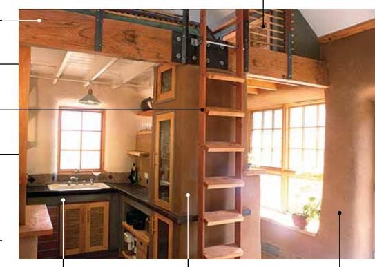
Wood-frame cabinet has an earthplaster finish on top. This transitions into an adobe thermal mass wall facing the south window.
